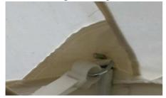
Additionally, the 6 guy points on the side must be reinforced with a second triangular piece of canvas, 300mm in length (one side), sewn to the edge of the eave with the point extending into the roof section.
